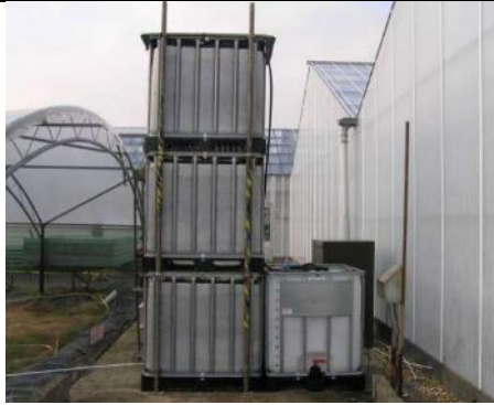
Figure 3: Biofilter system. Courtesy of the Voluntary Initiative (2013)
