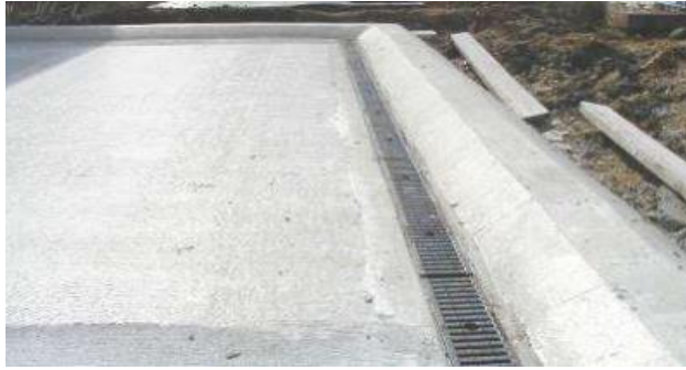
Figure 1 Concrete pesticide handling area. Courtesy of the Environment Agency.
